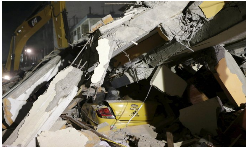
Earthquake damage in Ecuador. www.thehindu.com
